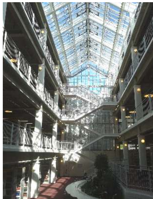
[Photograph 9] The restructured building
