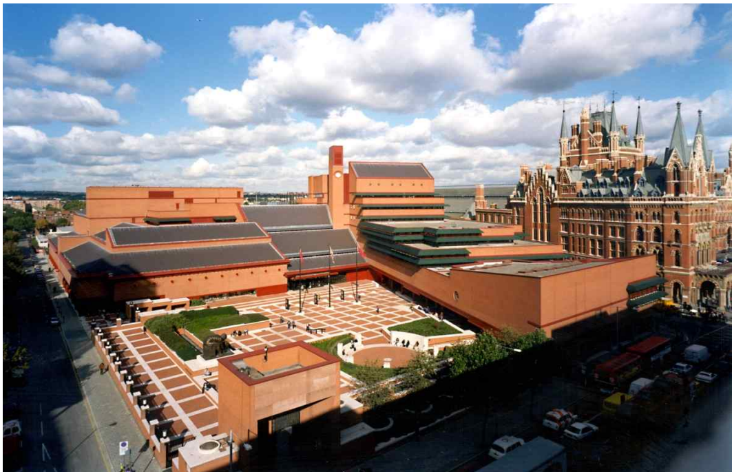
[Photo 1] The British Library site at St Pancras, London
